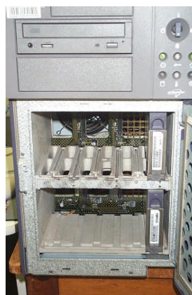
Server with hard-disks partly removed for cleaning; casing decontaminated and dried on site in mobile drying chamber
