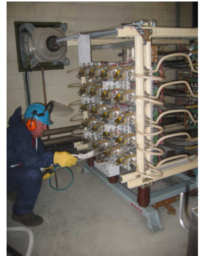
Dry Ice Blast Cleaning of soot contaminated Thyristors
