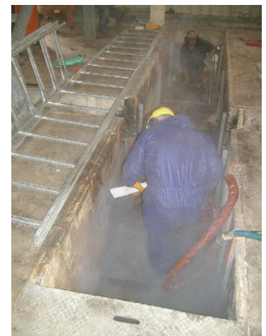
Dry Ice Blast Cleaning of floor recessed cable trenches
